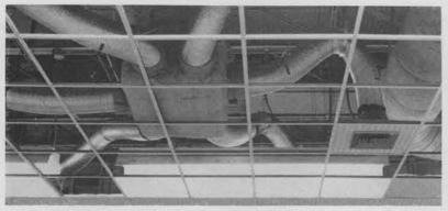
SPIDER-LIKE, the giant air conditioning ducts above the 705 computer spread out behind a false ceiling. Seven units move 2,000,000 cu. ft. of air hourly to provide constant comfort.
